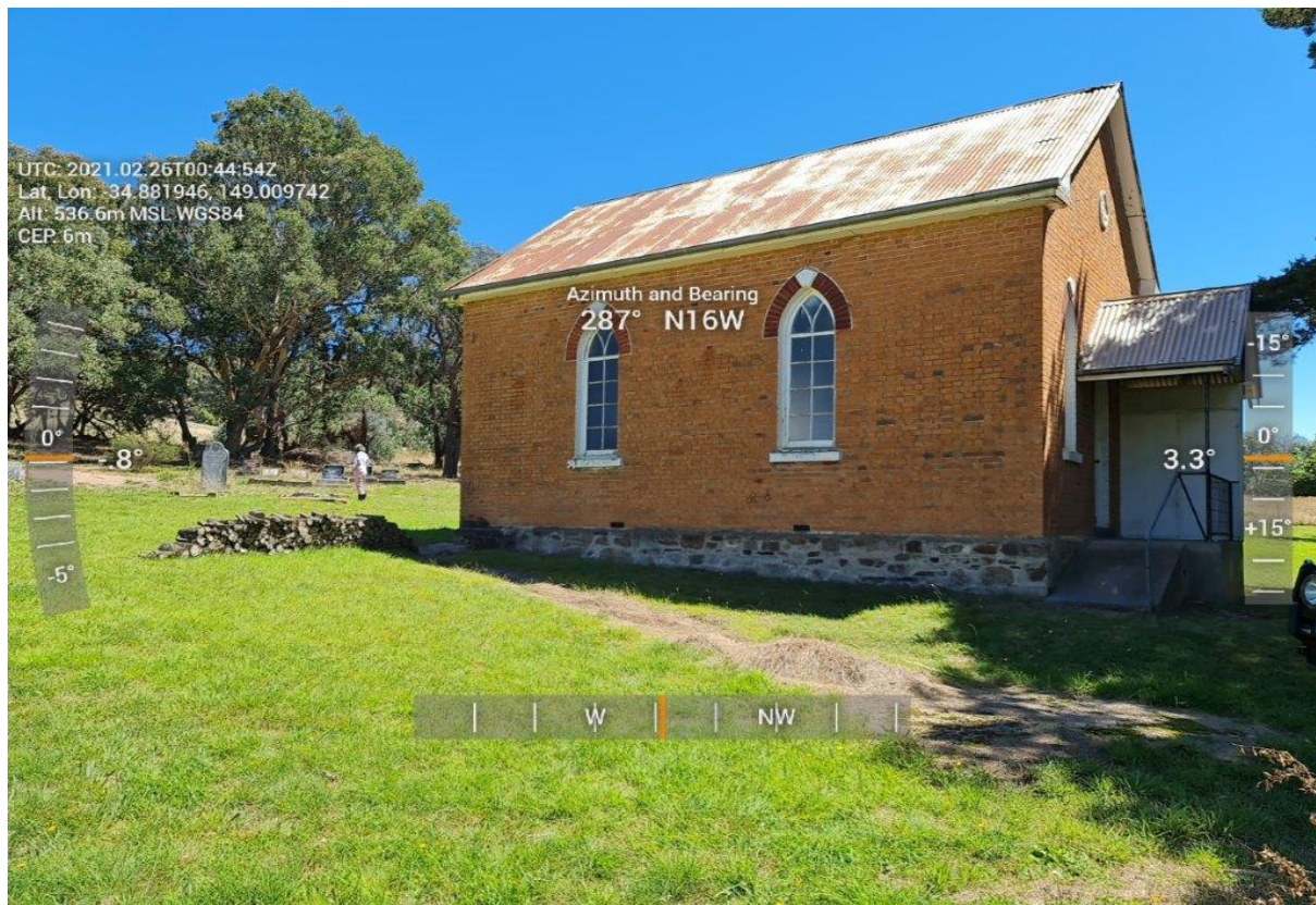
Figure 6: Existing chapel building
